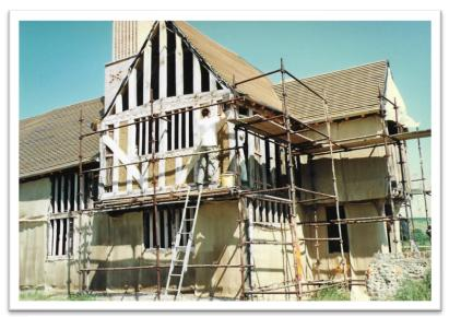
Pictured above: The studs repaired, wattle fixed, and the daubing being applied on the front by Andy.
